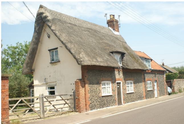
Old Timbers & Flint Cottage, Rickinghall
